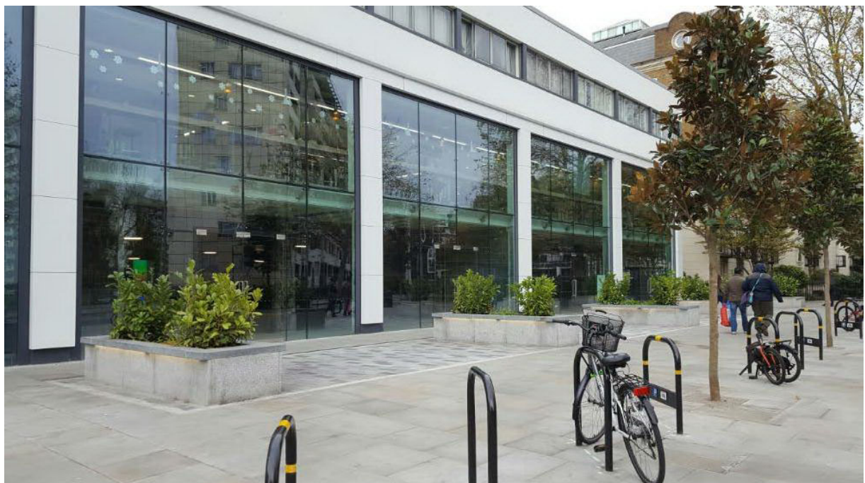
View of Bishop's Bridge Road frontage (Units 4 and 5 are the two left hand glazed frontages).
